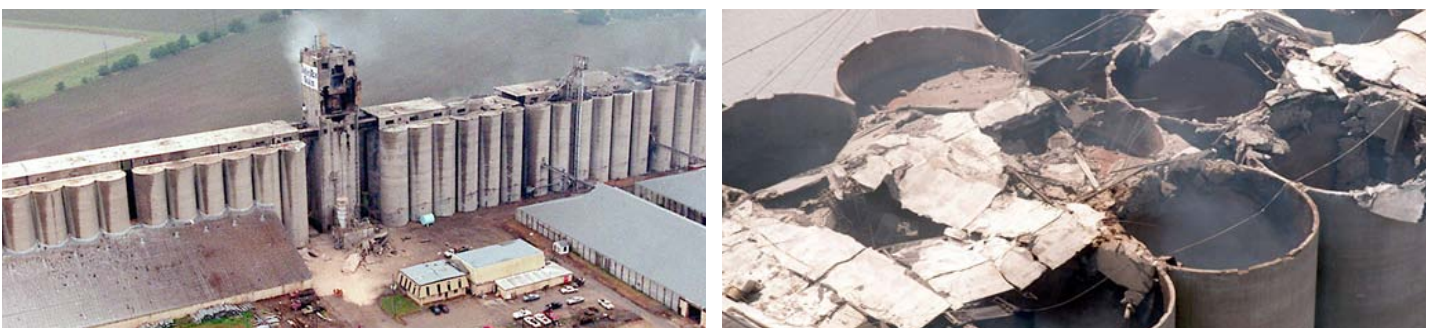
Figure 8. View of the DeBruce grain elevator after the explosion (upper gallery on right)
