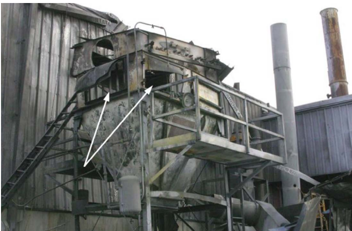
Figure 3. View of the dust collector (outside) and the facility (inside) after the dust explosion
