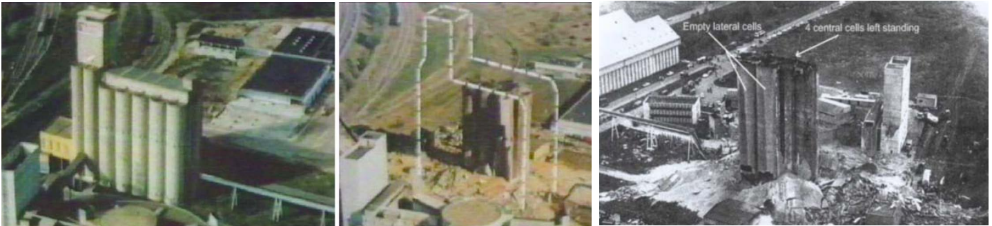
Figure 6. View of the Metz grain elevator before and after the explosion
