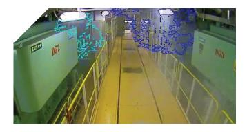
Fike Video Management Software is used for detection configuration and simplifies annual testing using computer based software routines.
